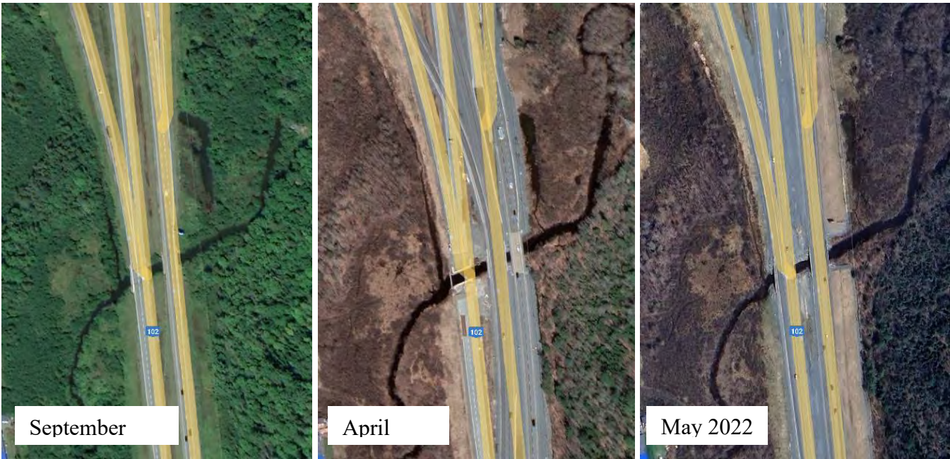
Figure 13 Temporary realignment of Hwy 102 at Site 2.
